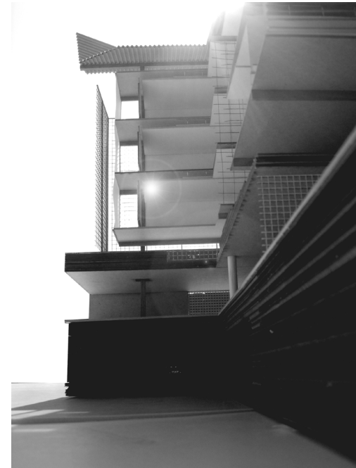
Fig. 72. View of classrooms along the west side.
